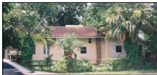
This vacant home is the future proposed site of NJCDC's office and community meeting center.
